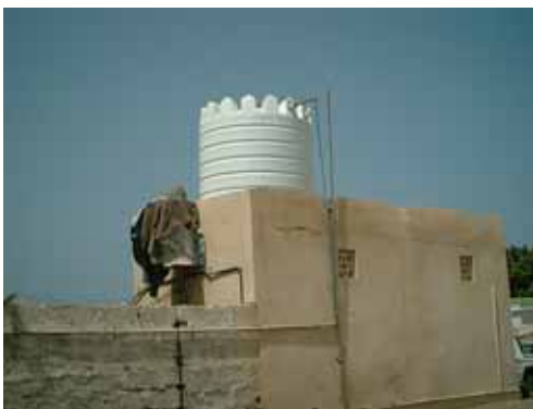
The Water Tank Positive for V. cholerae
